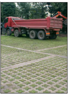
TYPICAL GRASSCRETE PAVING AFTER INSTALLATION
