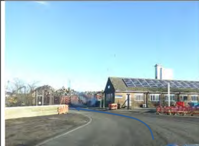
8.4.1.3. – View at crossing
