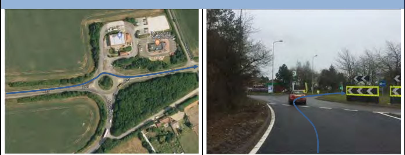
8.8.3.1. – Aerial View of Location 8.8.3.2. – View of entrance to roundabout
