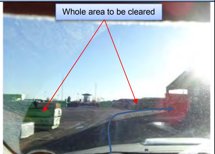
8.4.3.2. – View prior to bend
